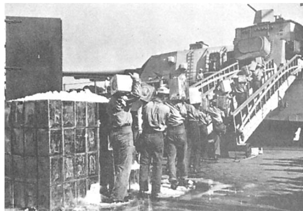
Figure 4-3.—The gangplank is an inclined plane.
