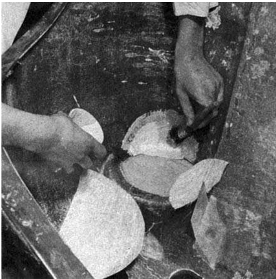
Figure 16.39 Applying chopped strand mat
