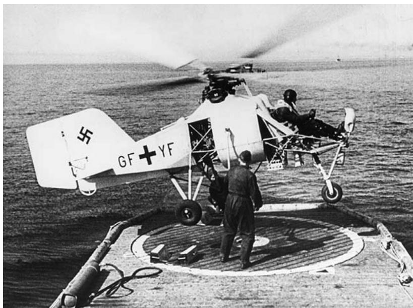
Figure 7.1-4 The Flettner Kolibri (Hummingbird) was the first synchropter and was an advanced and capable machine. Kaman developed the concept and produced the successful Husky and K-Max models. (Steve Coates.)
