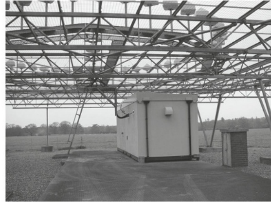
(b) Doppler VOR (DVOR) navigation aid (photo courtesy of T. Diamond)
